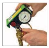
2L. Attach Charging Assembly (90.310.040 or 90.310.045) to the quick disconnect filler valve on the control panel.
