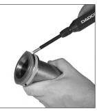
2. Remove the seal and piston rider. Pry the seal off the rod using the Port Servicing Tool, (90.320.8), be careful not to scratch the inside of the groove. Discard the seal and piston rider.
