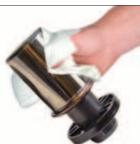
2. Lightly polish the rod surface with an emery cloth (600 grit). Inspect the finish of the rod for any scratches or gouges. If the rod is damaged it must be
